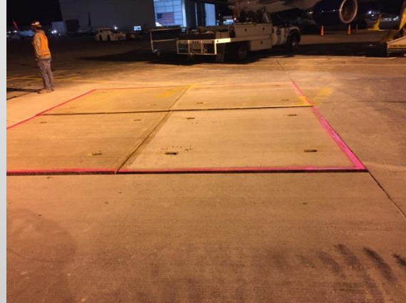
Airfield Pavement Replacement
